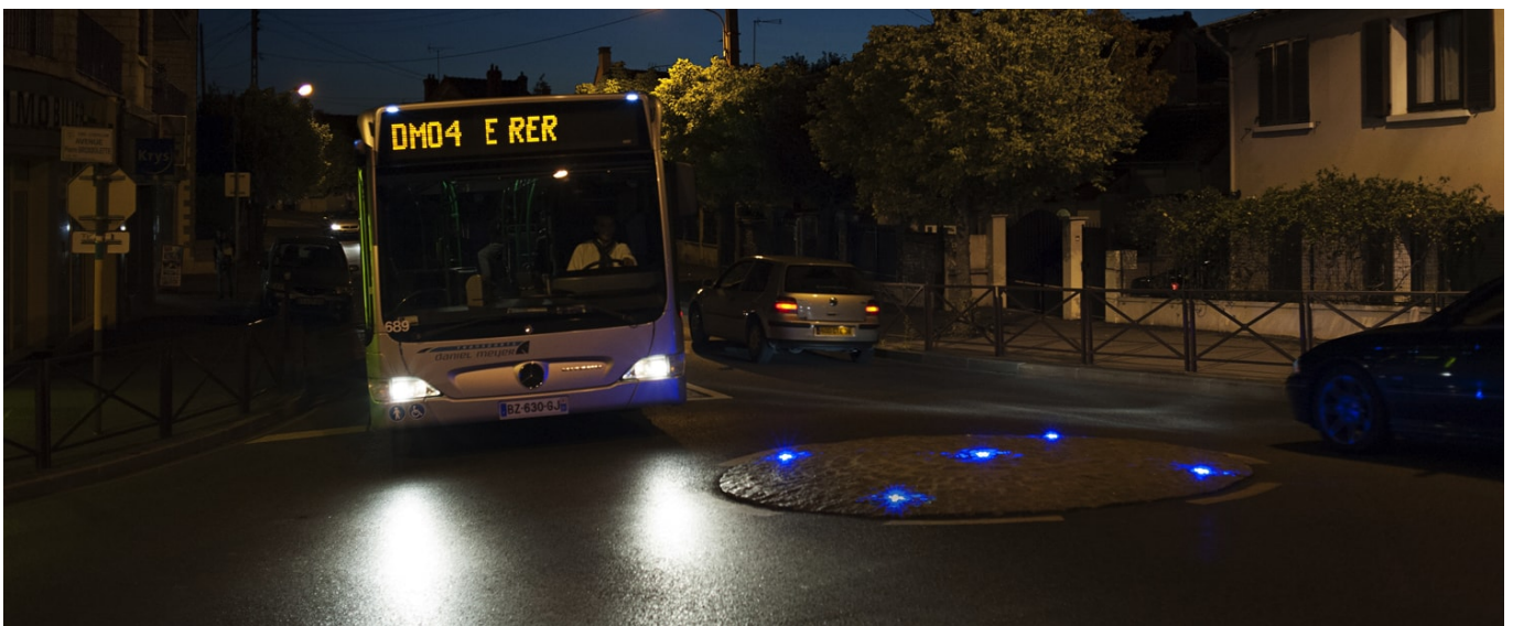
Mini-roundabout. Security marking on a vehicle-proof mini-roundabout in the city centre of Viry-Châtillon. Extra-low voltage embedded road beacon ECO-870 (constant markup with 24 blue LED visible through 360 degrees). Photography : Karolina Samborska.
