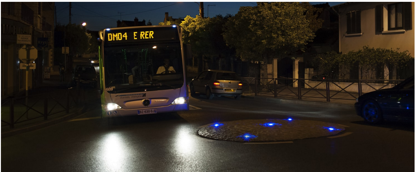
Mini-roundabout. Security marking on a vehicle-proof mini-roundabout in the city centre of Viry-Châtillon. Extra-low voltage embedded road beacon ECO-870 (constant markup with 24 blue LED visible through 360 degrees). Photography : Karolina Samborska.
